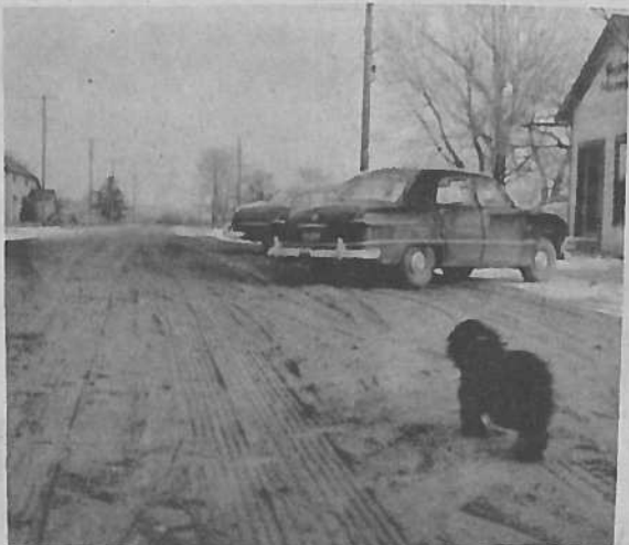
Nottawa Township spreads gravel where needed in east half of Weidman. Shown above is East Main Street, formerly under water each time it rained. Now it's good parking.
