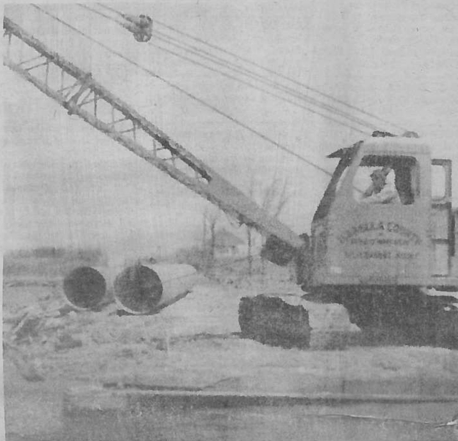
BIG MACHINES ON THE MILL POND ROAD have been busy since last weekend, preparing the north road for blacktopping after the further north stretch is done. Shown above is the big crane which prepared the pond-bottom and set in two giant tubes replacing the dangerous old bridge at that point. Fill trucks and graders have been working since Monday on widening the pond road, raising it, and creating a two-way area at the corner of the pond road and the Air Line. Needless to say, Weidman folks are jubilant.
