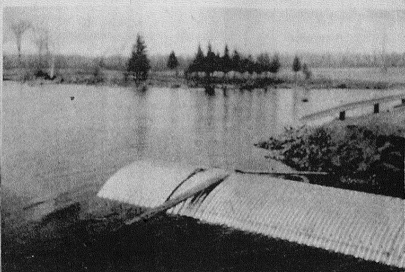
NORTH ROAD REBUILT AT OLD BRIDGE SITE. --Upper right shows the size of the new steel tube installed last weekend, replacing the small ones which washed out in the recent failure of the road's construction at that point. Lower left shows the crane nudging the steel tube into position. Larger pictures, upper left and lower right, show the depth at which the new tube was installed. Messenger Photos.
