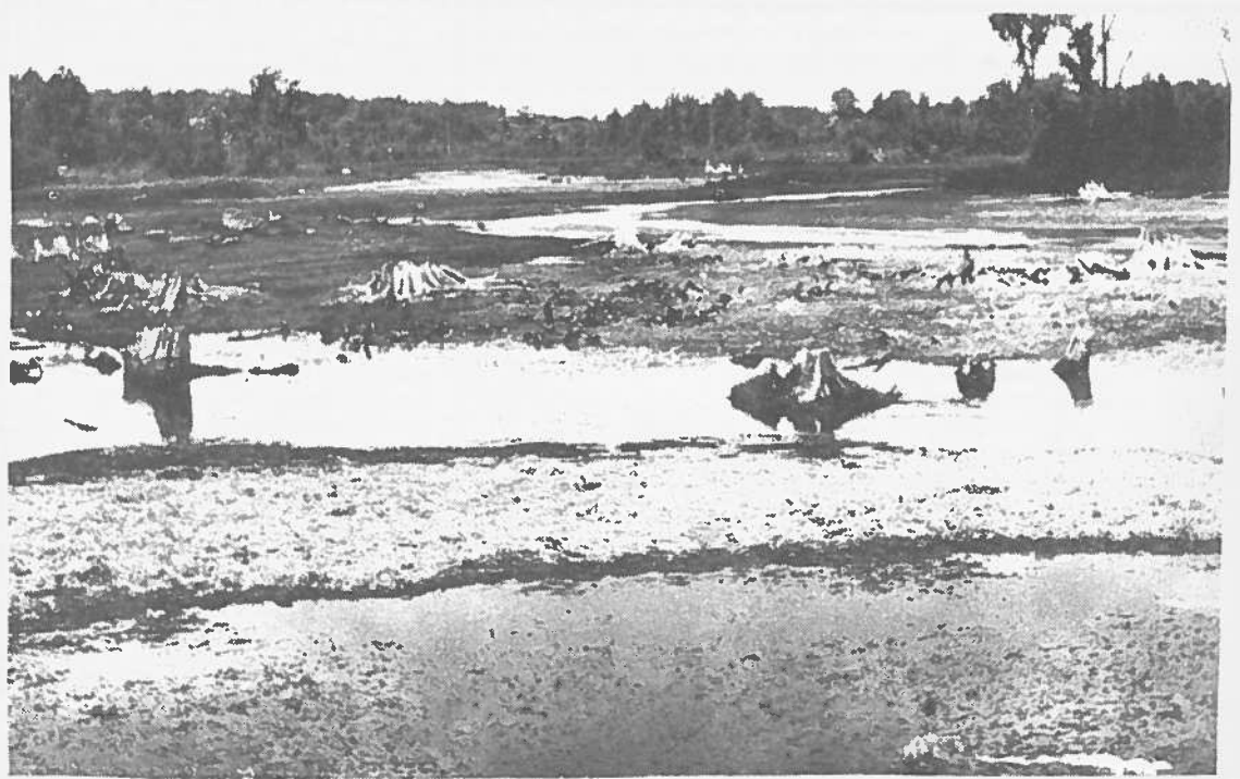
THE WEIDMAN POND WAS DRAINED--To allow a resort developer to see what the bottom looked like. It looked like this, only worse on the eastern section, or looking north from the mill. The above photo, by Meryl Graham, is a view from the north road, or the western section of the east Pond. Obviously, the Pond's bed was the remains of a cedar swamp when John S. Weidman put in his first crude wooden dam to hold logs for his sawmill, back in 1893. The dam has been rebuilt a couple of times since, of cement and steel, but the bottom of the Pond remains as the day John S. started backing up waters of the Coldwater River and Walker Creek. The resort promoter, Douglas Hollabaugh, of Lansing, hopes to make a beautiful lake of the east section of the Pond. We hope he does! He proposes to clean out the stumps and debris, deepen it, and subdivide land.
