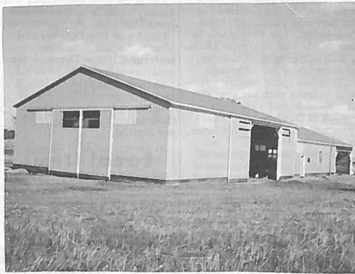
WEBER'S SAWMILL HAS SPANKING NEW PLANT --Above is the 50x128-foot new building of Weber Bros. Sawmill a mile north of Beal City. It's an imposing building, finished in steel corrugated turquoise-blue siding and plenty of space inside to house the mill's automated machinery plus a new log peeler from the Morbark factory at Winn.
