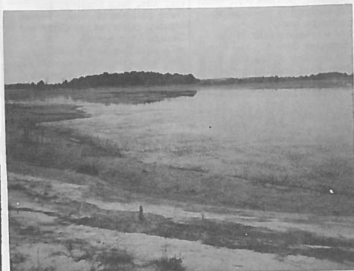
THE BREAK IN THE DIKE WAS NOT REPAIRED, and the Mill Pond was drained--again. Fishing was just beginning to pick up at the famous old Pond, after two years of undisturbed water depth. Above Messenger photo was at the east side of the Pond, at the Mill. That's a mess of weeds you see here, with some pools of shallow water in places in the Pond. But it is drained.
