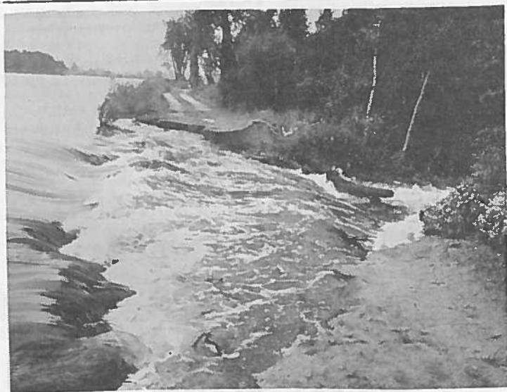
DIKING ON THE EAST SIDE OF THE MILL POND GAVE WAY-- in two places, one around the point from the above photo, sending tons of water rushing into the Scut Drain which runs along the mill road on the north side, crosses under the road and empties into the Coldwater River below the dam. Cottagers at Coldwater Lake suffered doubly because of this break in diking.
