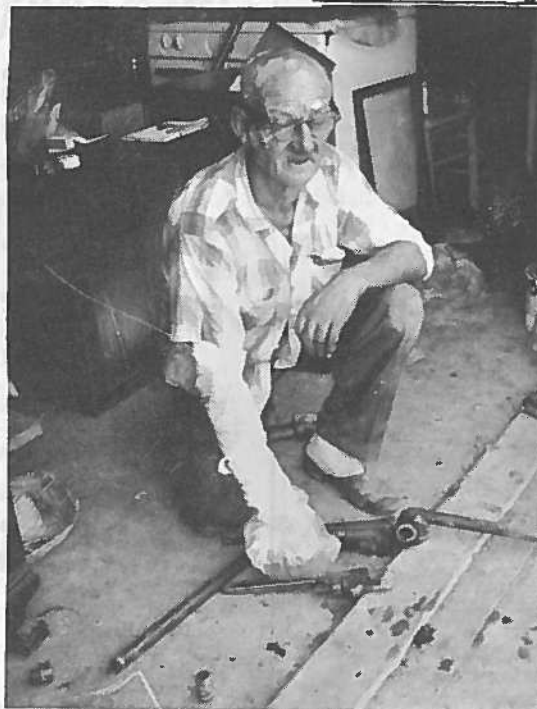
CLARENCE GEITMAN WORKS ON PIPE FITTING FOR WATER--Above photo shows Clarence Geitman as he worked in his rubble-strewn garage attached to his wrecked house. Sunday he was attempting to repair his water-well line, he told the Messenger reporter. He suffered burns on his arms, right hand, leg, and head and face. Scalp burns show in the photo.
