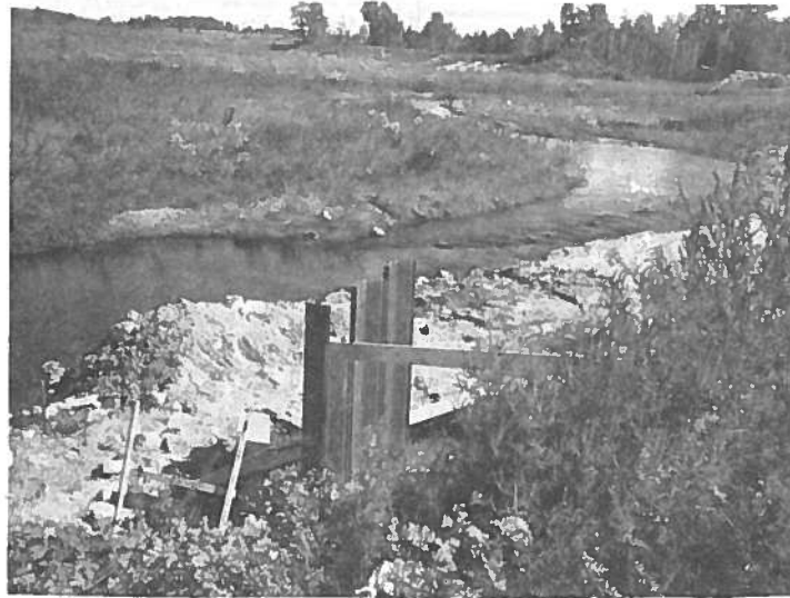
THE START OF THE NEW DAM--At the Mill Pond, which will be of steel and cement construction of the nature of the dam at Lake Isabella, that is, self-controlled. The dam site is a few feet north of the old dam, which will be used for expelling the water under the road. Allen Lumber Company is doing the steel work. Messenger photo
