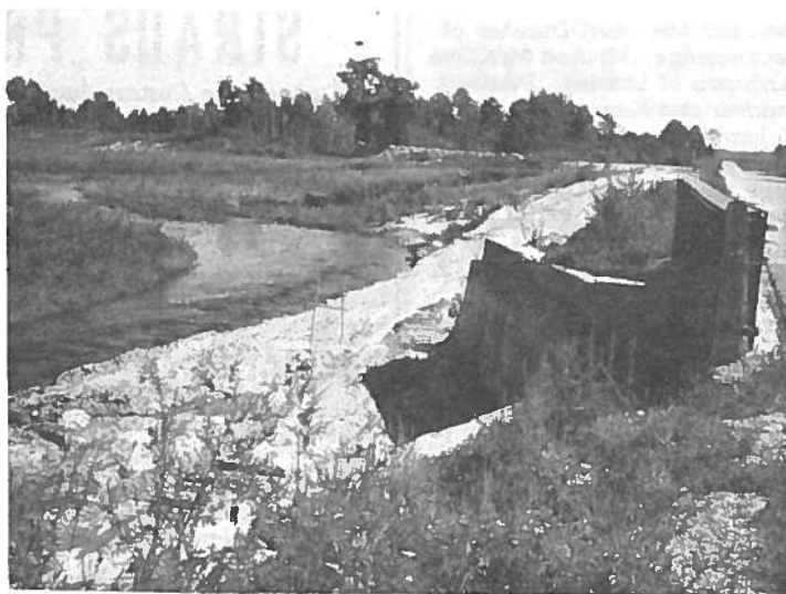
ANOTHER VIEW OF THE DAM SITE--At the Mill Pond. Shown above is the old dam as it sits, with land fill in front of it and the Coldwater River meandering off in the left and upper part of the picture. Messenger photo
