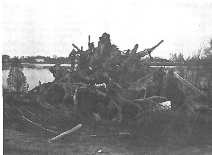
PART OF THE DEBRIS HAULED OUT-- Of the west side of the Pond by the big crane. The road was not closed, but autos ventured cautiously into the swirling waters; and many had wet brakes afterward, though no accidents were caused by the condition of the road. The water had gone down by Sunday, and the road was clear, though heavily damaged. Twenty-two roads in Isabella County were reported seriously damaged by flood waters after the heavy electrical storms. Messenger photos
