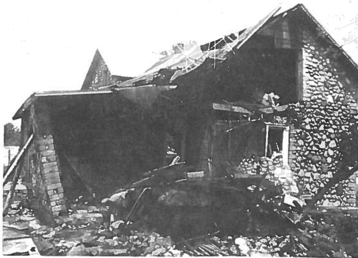
THE WILLIAM MIKOLIC HOME WAS NEARLY DESTROYED --By an explosion last Friday, believed to have been caused by leakage of propane gas. The home is located northwest of Brinton, just off Bawkey Road, west. At 10.30 the Nottawa and Sherman Fire Department responded to a call and found the wreckage but little fire. The family used 200-pound propane gas cylinders, considered small containers. Miraculously, no one in the family was injured, though two members of the family had left the explosion area seconds before the blast. The state fire marshal investigated for cause. Messenger photo
