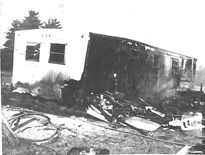
THE WEST END --Of the trailer home on the Melanowski place was the most burned-out in Saturday's fire, but the family said the whole structure was burning, from one end to the other. Straw packed around all sides of the home, and underneath, appears to have been quick fuel to the flames of undetermined origin. A $50 grocery purchase, newly made, burned up. Messenger photo
