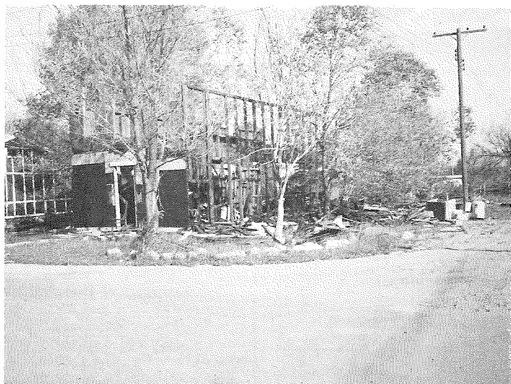
THE OLD ROY GREEN HOUSE--At the corner of Main and Second Streets on the east side of Weidman, has been cited as a hazard that might be dangerous to children, and also as an unnecessary slum-spot that brings down valuations of every home in the neighborhood. Above photo was taken early last autumn. Messenger photo
