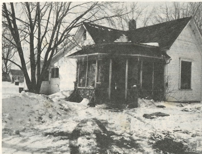
ONE OF WEIDMAN'S OLD LANDMARKS-- Was practically destroyed by fire last week. It's the old Neil Faling house, occupied in modern times by Muriel Miller and her family. The Nottawa and Sherman Volunteer Fire Department did its best, but the structure of the house--built by a master craftsman--was such that it was difficult to locate the source of fire. The Neil Faling house stood these many years, the craftsman's work standing up through the ages.
