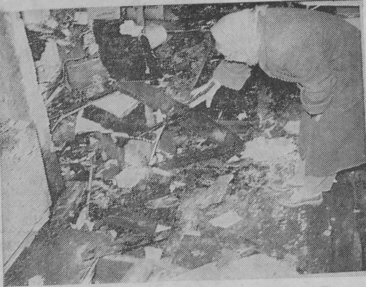
RUBBLE REMAINED of the compact office, pasteup and photographic departments of the Messenger after Sunday's fire. Origin of the disastrous fire is believed to have been either the oil heater or the chimney.
