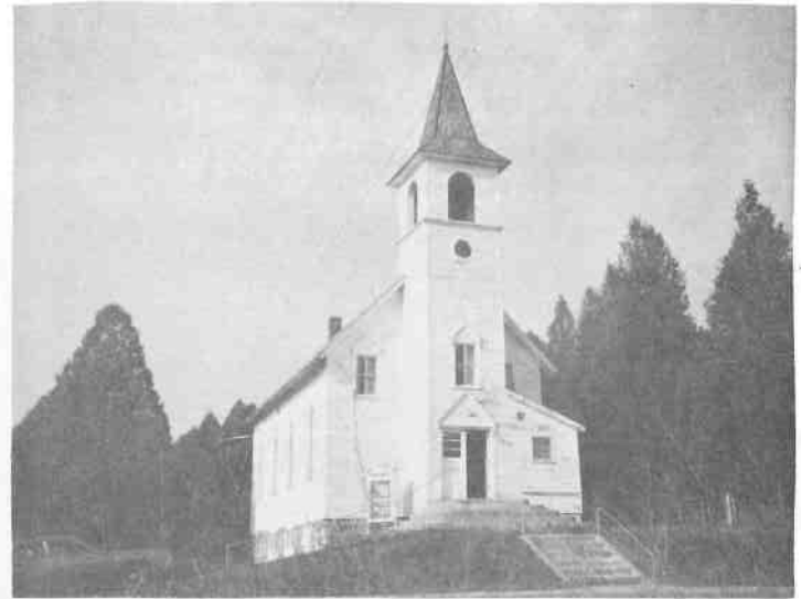
THE OLD LUTHERAN CHURCH IN BROOMFIELD--Was built in 1894, and has no conveniences for Sunday School rooms and other details considered necessities today. The entire congregation of 35 families is active in the plans and work of building the new church. Messenger photo
