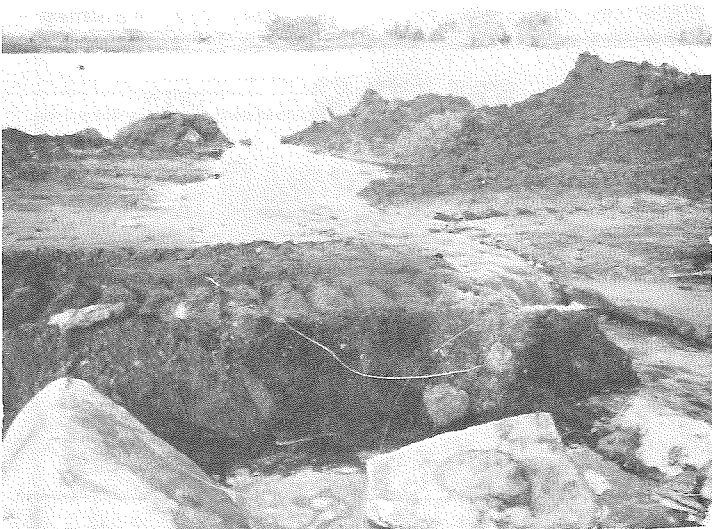
HERE SHE COMES! --This is how the emergency spillway on Lake Weidman operates. The spillway area is reinforced with steel casings deep down into the ground, to insure prevention of washout of the spillway area. Messenger photos
