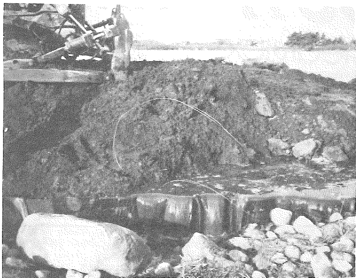
SPILOVER BEGINS AS A SMALL OPENING --Was cut at water's edge to allow the lowering of water level in Lake Weidman.
