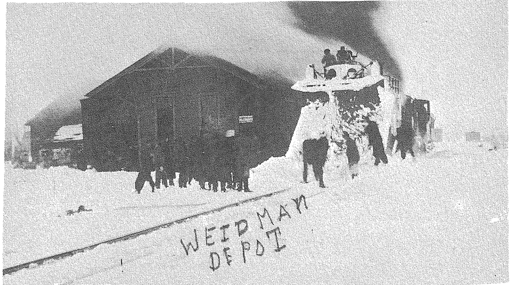
THE BIG SNOWPLOW WAS CALLED IN TO GET THE ENGINE AND TWO CARS BACK ON TRACK--At Weidman, in the 1920s. The "big snowplow" probably was no bigger than our present road snowplows, but it was the world's wonder to us at the time. The "big snowplow" was called to right the derailed cars and engine because of its superior size and engine power. Photo sent to Mrs. Melvin Loeding by the widow of Ernie De Hart of Coalmont, Tenn., who was a former Weidman resident. The old pictures will be placed in the Weidman Library.
