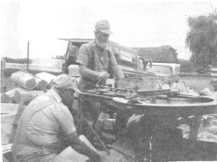
AND HERE'S LYNN MIX OF HASTINGS--Who brought his ancient shingle-cutting machine up for the work-bees at the Sherman City Church. It's a remarkably simple but efficient gadget, taking blocks of cedar wood and shaving 'em off into perfect shapes for roof shingles.
