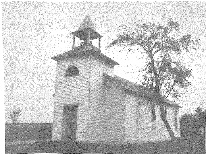
THE BELFRY OF THE SHERMAN CITY UNION CHURCH--Is now re-installed, having first been rebuilt with finishing touch of the intricately-cut shingles shown above. Wilbur Wright did the artistic job with a jigsaw in his special workshop.
