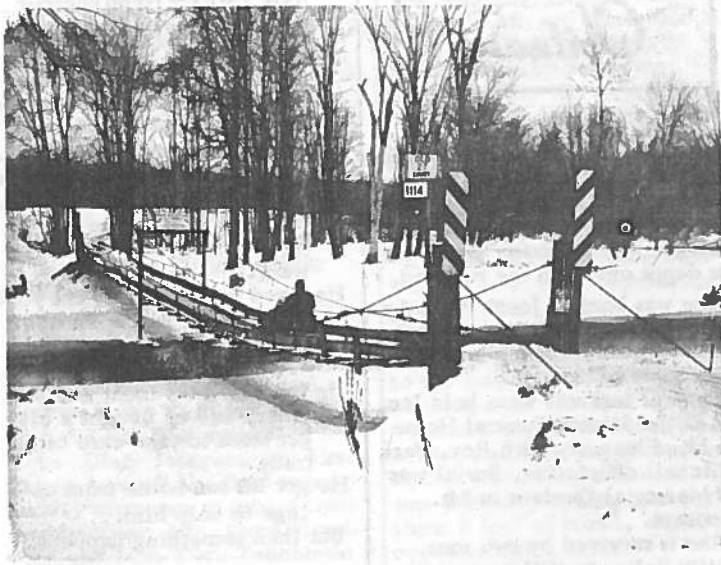
THE LITTLE MAC BRIDGE --On the Elwood Miller farm, where the third annual Lil' Mac Bridge Day will take place Sunday, Feb. 16. The bridge was built by friends and neighbors of the Millers--and the Millers--for snowmobile access across the Chippewa River, and it is pretty much of a marvel of suspension-bridge construction, in a miniature way. This year there will be a "walk across the bridge," in the manner of the famed annual walk across Big Mac at the Soo; there also will be many winter scene enjoyments, and a great big hog-roast dinner.
