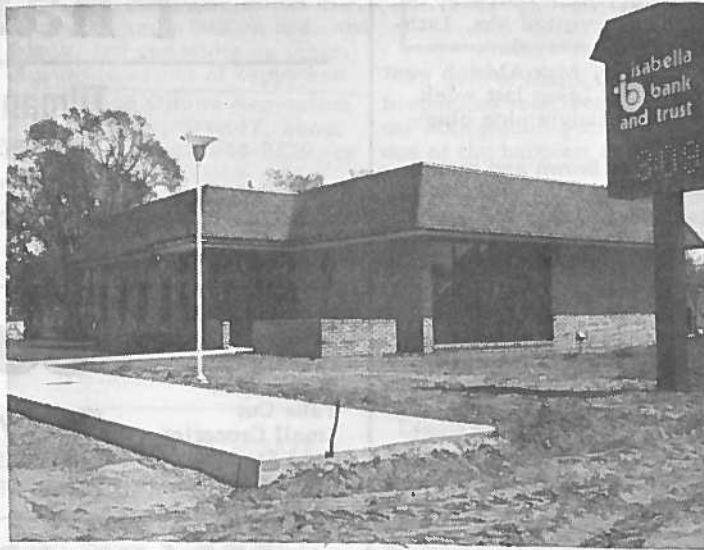
THE NEW BANK BUILDING IS COMPLETED--And only landscaping and paving remained at the time this picture was taken (last Friday). The Weidman Branch of Isabella Bank and Trust will open for business in the new place next Tuesday, May 27, and an Open House will be held Saturday, May 31, from 10 a. m. to 2 p. m., with bank people showing visitors all through the new building, its offices and its many unique facilities. Next Monday at the opening, at about 8.30 a. m., a ribbon-cutting ceremony will be a feature of the new bank's official occupancy. The public is cordially invited. Messenger photo
