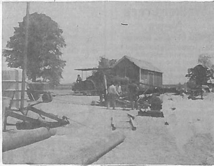
THE FIRST SAWMILLS LOOKED LIKE THIS--As shown during the recent Beal City Area Centennial celebration. The sawmills were crude portable contraptions with no safeguards for workers. Take a look today at Weber Bros. mill at Beal City or Maeder Bros. mill at Weidman, and you'll see sawmills still going strong, but in the modern manner. Messenger photo by Bud Fredrickson and Red MacLean of Mt. Pleasant.
